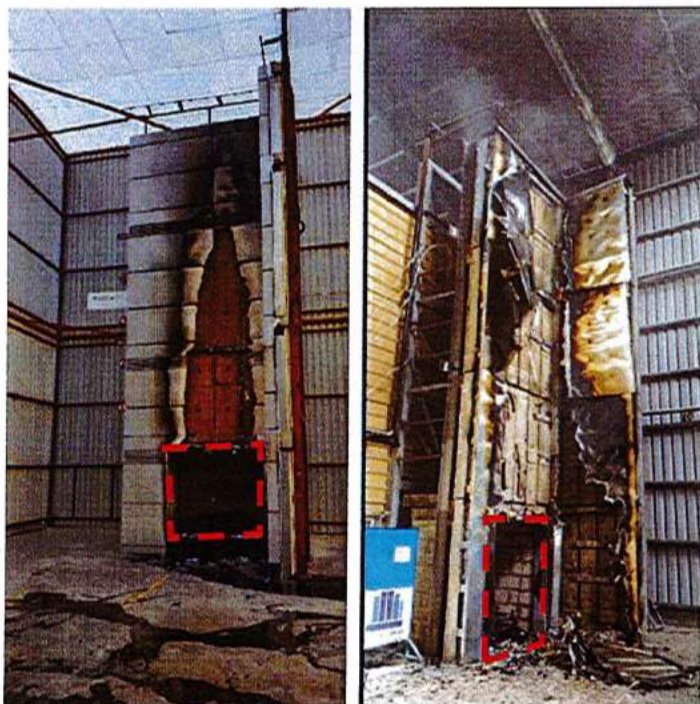
Figure 2 Comparative effect of the presence of cavity barriers adjacent to solid aluminium panels
